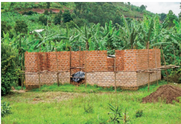
a house under construction with bricks itafâri 5, amatafâri 6. No.270
